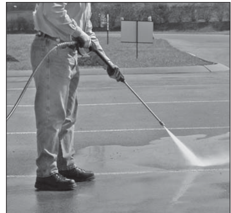
Figure 14 - Optimum angle to cleaning surface
