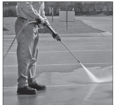
Figure 22 - Optimum angle to cleaning surface
