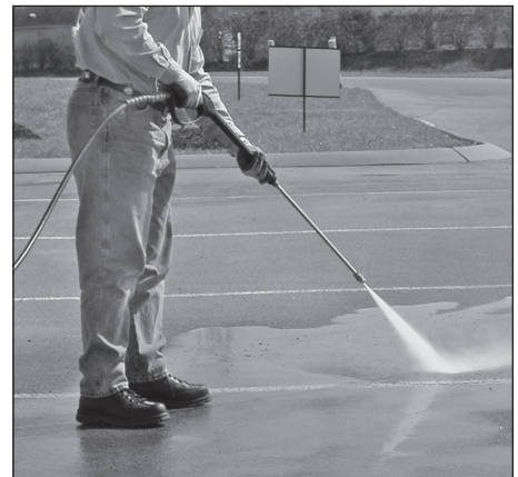
Figure 18 - Optimum angle to cleaning surface
